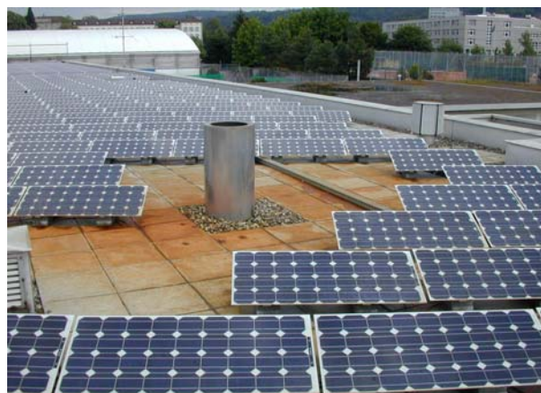
Fig. 19: Detail of a module edge close to a chimney.
